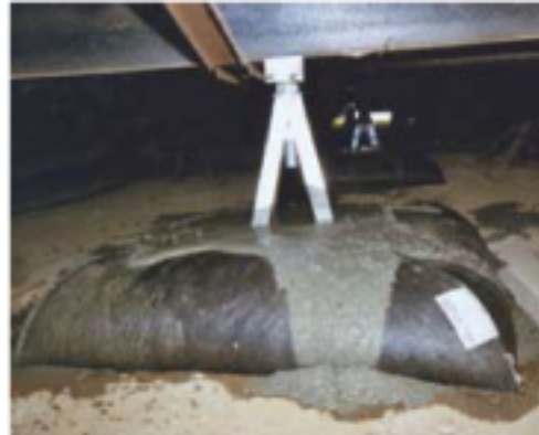
Close-up shows how concrete completely fills the geotextile bays and seeps through the bottom to form a concrete connection to the earth.
