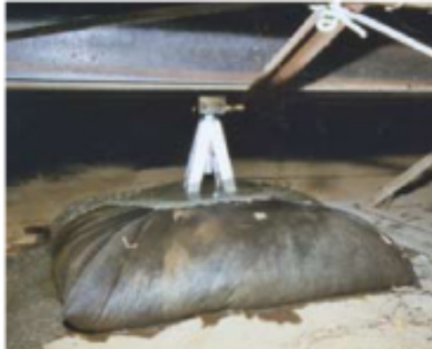
The concrete fills the bag forming a solid concrete attachment measuring approximately 6-1/4 sq. ft. At the right one of the temporary supported jacks is seen which is utilized to level and hold the home firmly until the concrete hardens in the permanent buttress system members.
